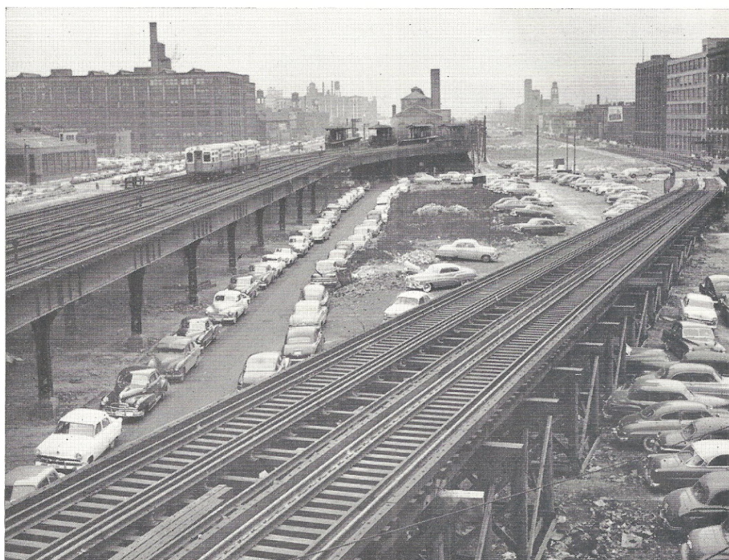
Incline to Elevated from Temporary Surface Track in Van Buren Street.
