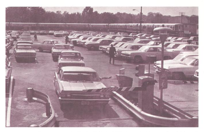
Improvements to the Congress terminal Park 'N' Ride lot initiated in 1966 with resurfacing, lighting, and stall marking, continued with the installation of electric gates and a hopper-type fee collection device.
