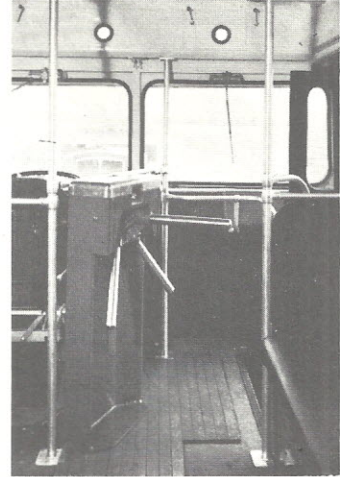
Bus Installation England
