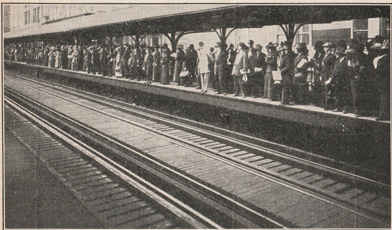
Photograph showing close tie spacing used on the Union Loop.
