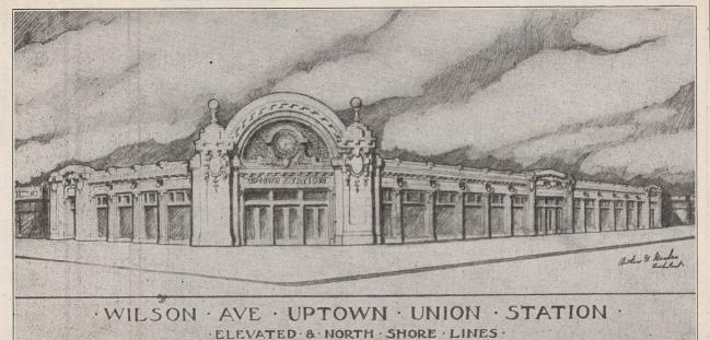
Work is progressing steadily on the new Uptown Union Station of the Northwestern Elevated and North Shore Line, at Wilson avenue and Broadway. It is expected to be ready for service by next April. The building has a frontage of 274 feet on Broadway and 112 feet on Wilson avenue. The plans provide for the building of a foot subway under Wilson avenue to connect the new station with the present one on the south side of the street.
