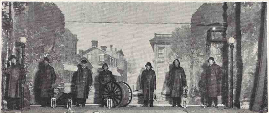
The Underground and Emergency Gangs
