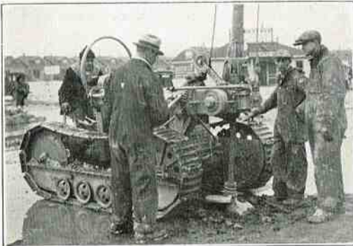
Starting To Dig the Hole for a Steel Trolley Pole
