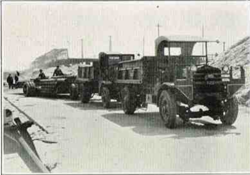
Hauling Trolley Bus Line Poles
