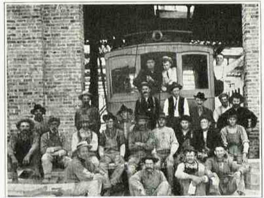
Group Picture of Some of the Men Engaged in Construction of Truck Shop Building at the West Shops in 1905. Reading from Left to Right in the Car: Charles Murphy, Deceased; Timekeeper Peterson, and Ed Plowright. Standing in Front of Car, Center, Edward Rafferty, Foreman and Wm. H. Figg, Superintendent in Charge of the Work
