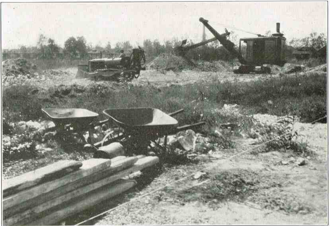
Breaking Ground for the New Service Station at North Avenue.
