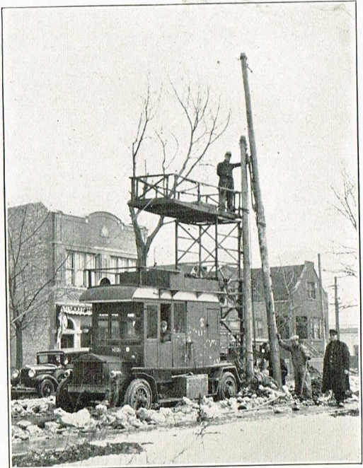
The Old Way of Setting a 32 Foot Steel Pole with a "Gin Pole"
