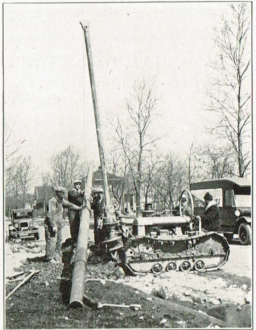
Setting a 32 Foot Steel Trolley Pole with the Earth Boring and Pole Setting Machine
