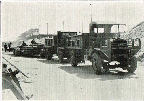
Hauling Trolley Bus Line Poles
