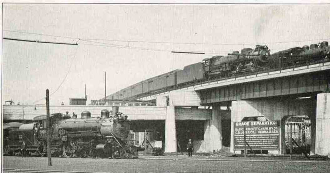
New Three Way Grade Separation at 16th and Canal—Burlington at Grade, Surface Lines on Canal Street Over Burlington, and St. Charles Airline Over Canal.
