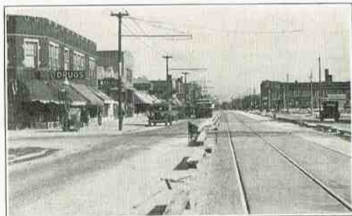
Finished Concrete Looking East from Meade Avenue
