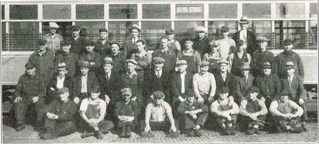
Burnside Pull-In Crew
