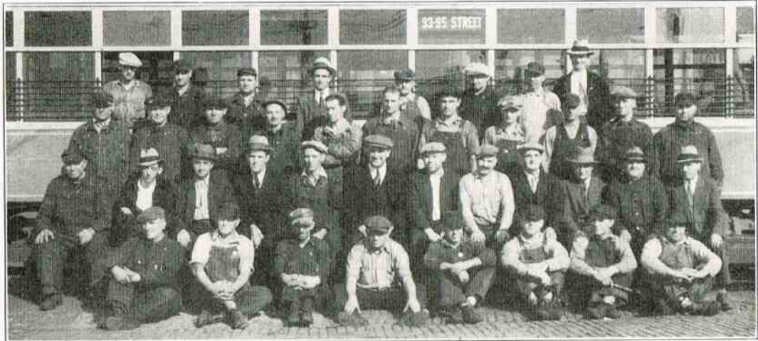
Burnside Pull-In Crew
