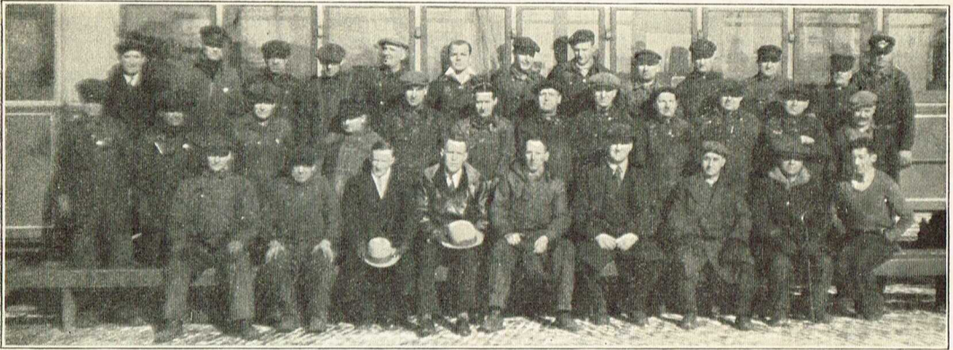
Burnside's Winning Repair Crew
