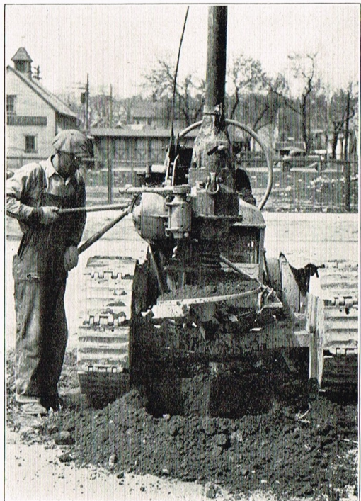
Pole Setting Machine Digging Hole
