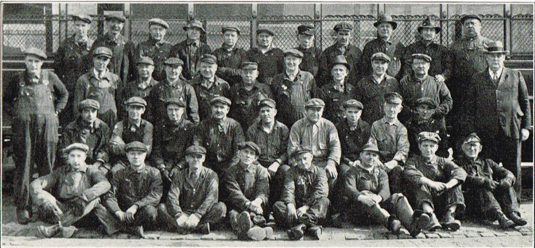
Cottage Grove Pull-In Crew
