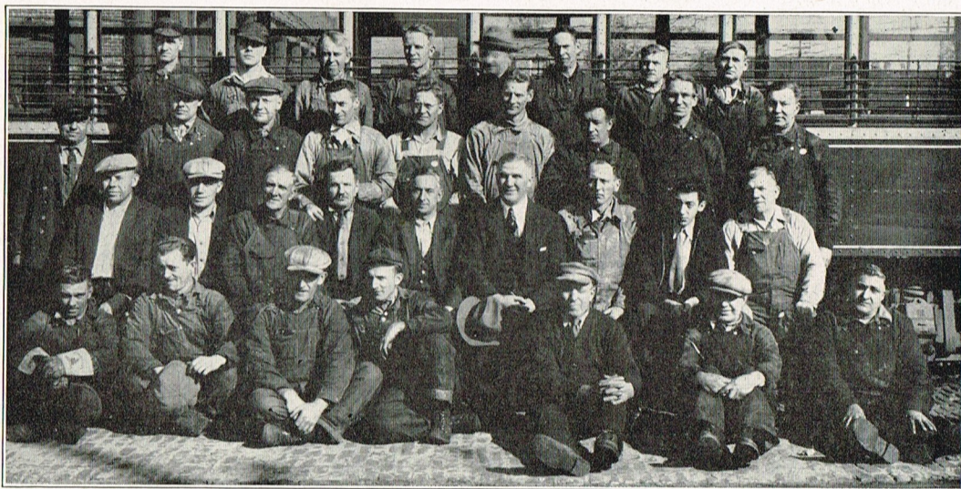
Burnside Pull-in Crew
