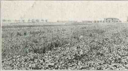
Cottage Grove and 79th Street in 1908
