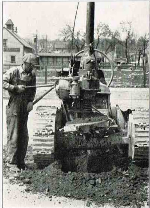
Pole Setting Machine Digging Hole
