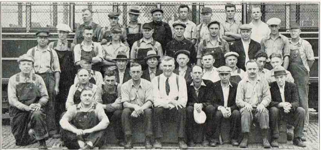
Burnside Pull In Crew
