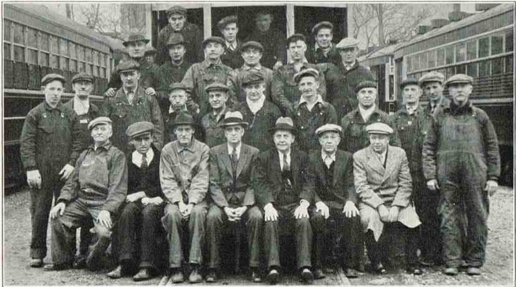
Elston Pull-in Crew
