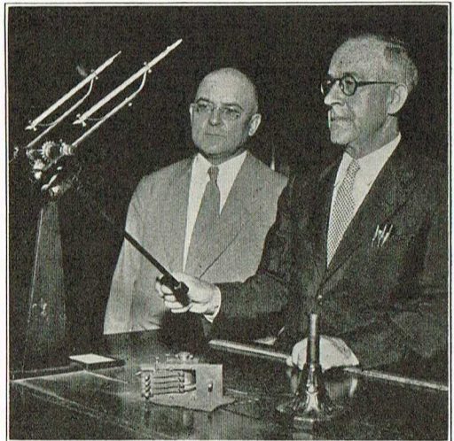
C. A. Donnel, Meteorologist, With Willis R. Gregg, Chief U. S. Weather Bureau, Using a Whirling Cyclometer.
