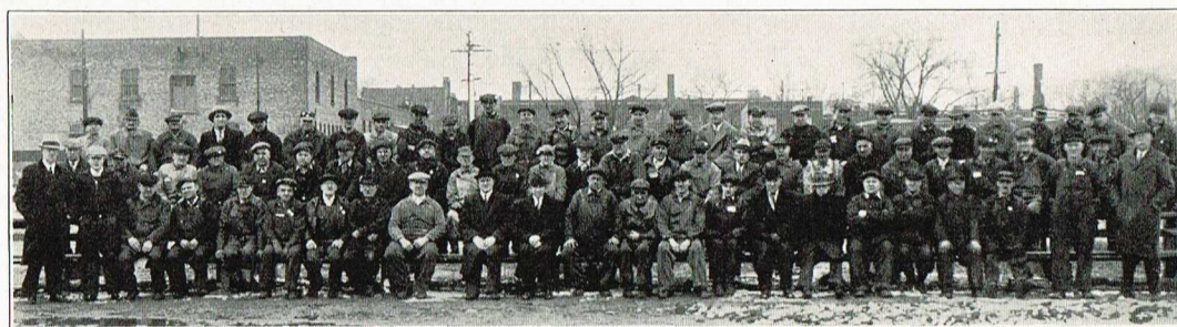
77th Street Pull-In Crew
