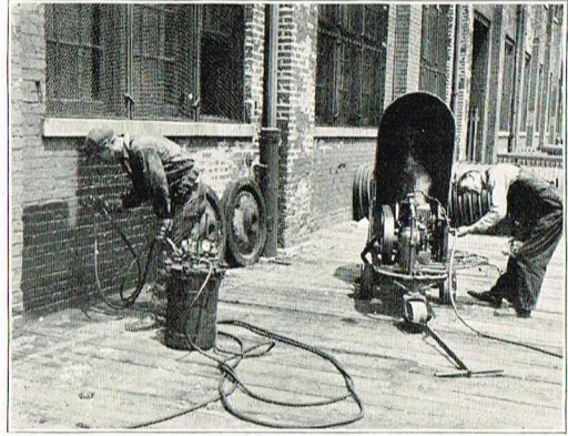
Spray Painting South Shops Buildings
