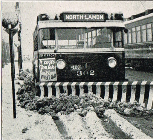
Detachable Trolley Bus Snow Plow Which Aids in Cleaning Streets of Snow.
