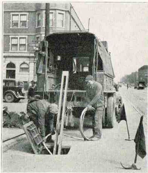
Feeding cable into conduit.
