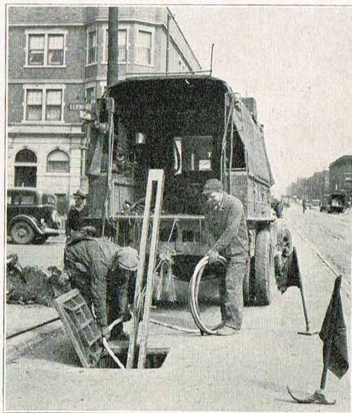
Feeding cable into conduit.
