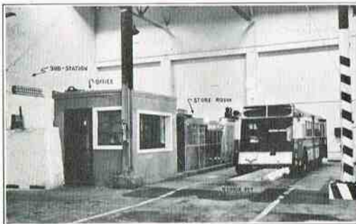
The repair kit, foreman's office and the storeroom of the new bus depot is shown in this shot taken at the rear of the north bay.
