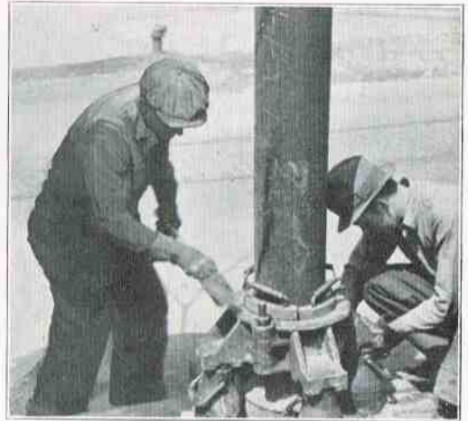
New pole-pulling method
