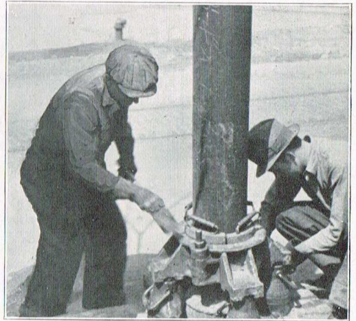
New pole-pulling method
