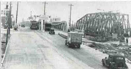
New Ashland Avenue Bridge
