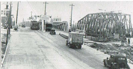
New Ashland Avenue Bridge
