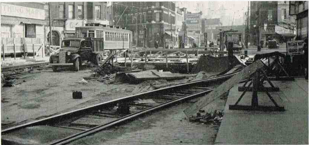
DURING SUBWAY MEZZANINE STATION CONSTRUCTION
