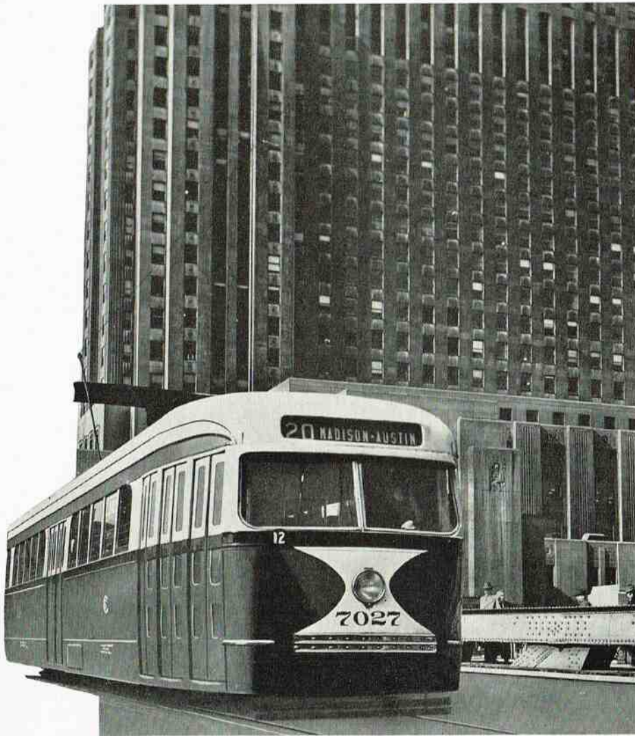
STREAMLINED CAR ON MADISON STREET BRIDGE
