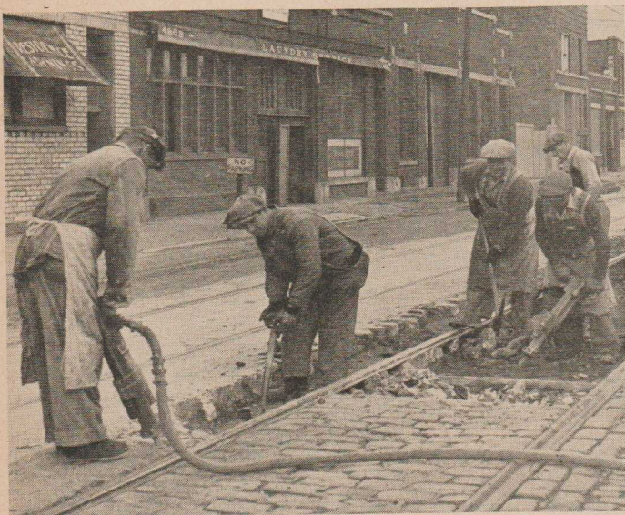
THE BREAKAWAY: Pneumatic paving breakers are used to dig out paving blocks and break up the concrete paving foundation, thus exposing the rail, fastenings and ties. After base of the rail has been exposed, the ties are tested (and replaced if necessary), rails renewed, surfaced and aligned, and new fastenings installed. The concrete paving foundation is then replaced and the track is ready for paving.
