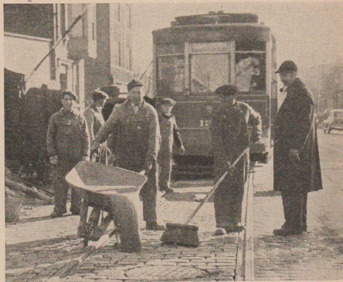
THE SMOOTHING: In paving the track, a bed is laid consisting of a layer of torpedo sand about 1 1/2" deep, and the paving blocks are then laid on this bed. Paving block is then covered with a thick grout (mixture of cement and sand) which is thoroughly broomed into the openings between the blocks and into the space under the head of the rail, and allowed to set.
