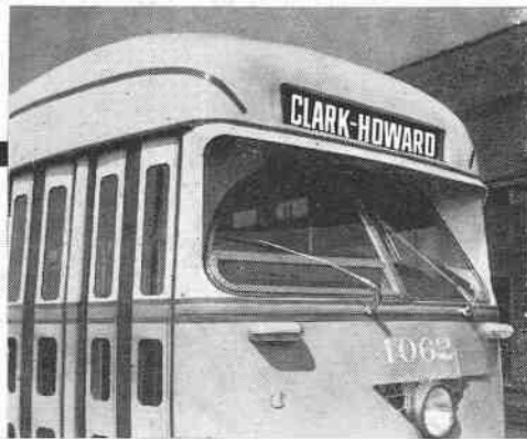
Clear vision ahead, with no night-time glare, is provided by new shadow-aproned slanted windshield.
