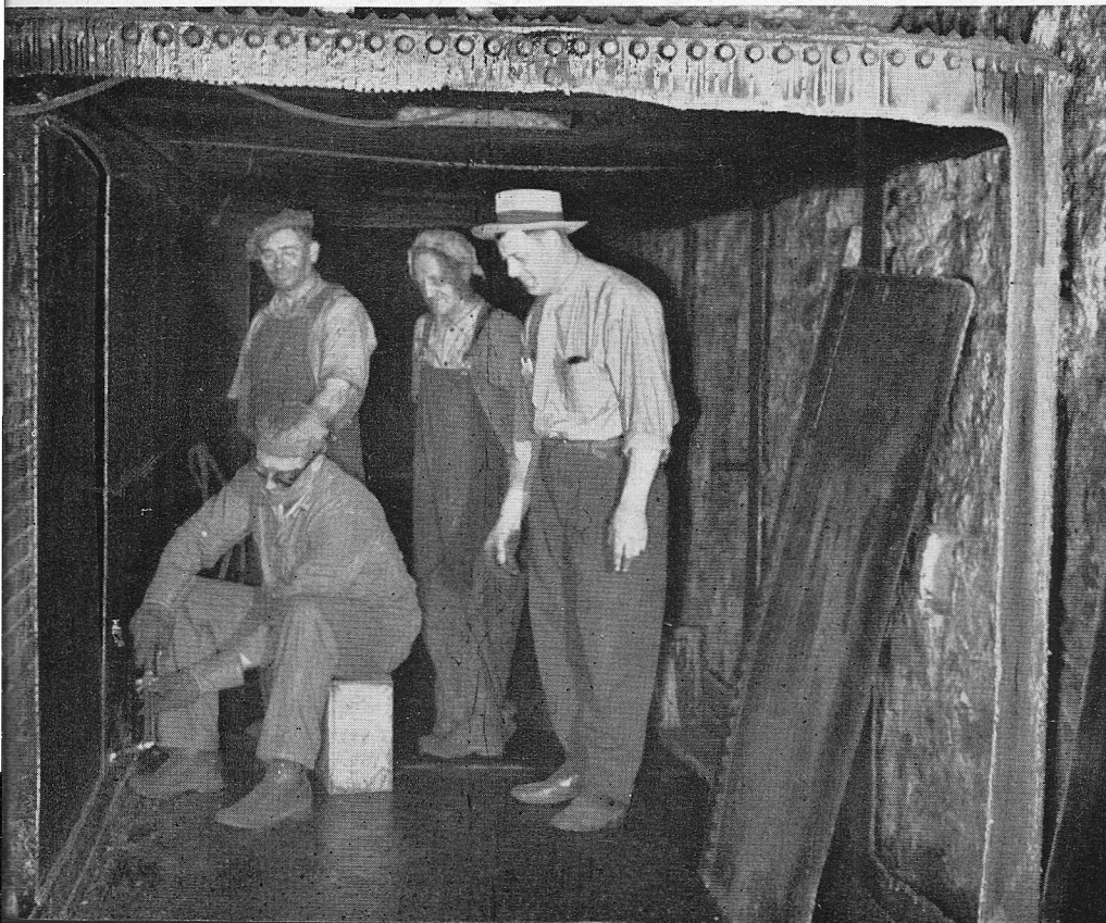
ABOVE —John Stacey and Frank Kozaritz cut an opening in the huge oil tank with a drill (note jagged edge) and air saw to prevent explosion. Ashes and sand on floor absorb excess slush.
