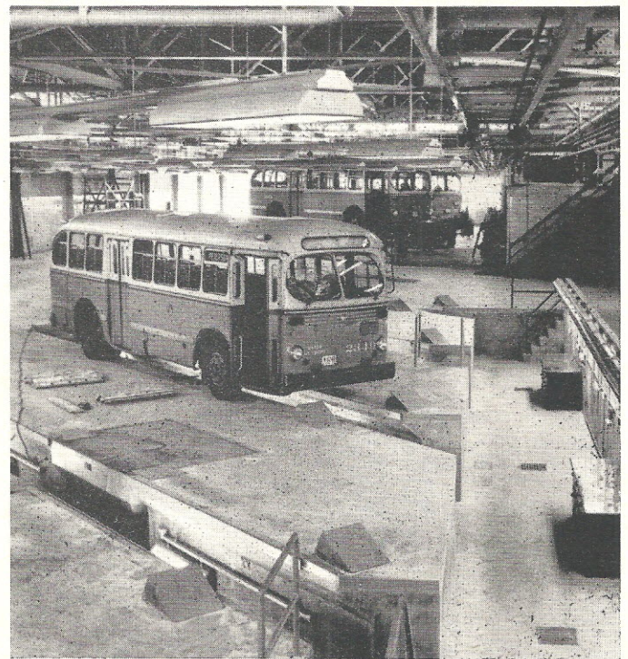
FOUR modern, well-lighted pits are available for repair work on buses. In the background are the five new bus hoists.
