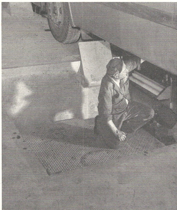
WORK pits in the service building are equipped with "levelators" used to simplify repair work in hard-to-reach places and to facilitate the removal of side-mounted bus motors.
