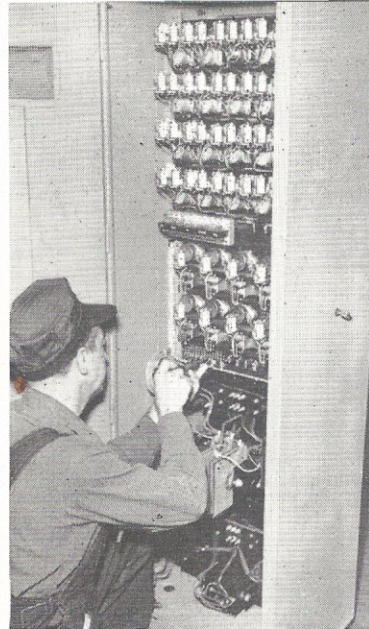
MOST of the electrical installation for line supervision was completed by CTA employees. Shown here adjusting the automatic timers is Electrician L. B. Farber .
