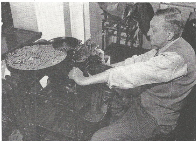
TOKENS are counted by this machine at the rate of about 2,400 per minute. It is usually operated by Nettie M. Kingsley, who was on sick leave. In her absence, Paymaster Tom Chamberlain demonstrated its operation. This machine is also used to put tokens into tubes for resale.
