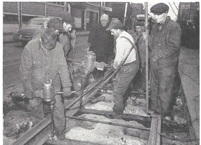
AMONG the many time and labor saving power tools used by Way and Structures men are these two—a tie boring machine, foreground, and a spike driving machine. This work was being done in connection with a large track renewal program on Clark street, near Sheffield.
