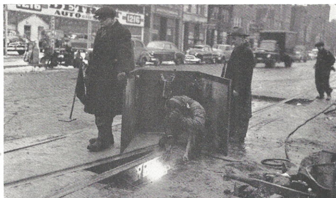
ELECTRIC welding crew restoring special trackwork on Western avenue near Division. Vincent C. Scimeca , electric arc welder, is welding in a new piece, replacing the broken arm of a switch mate. Frank Felski , left, is protecting the workman from oncoming traffic, and Tom Qualter , welding foreman, is observing the job. This type of welding is applied for repair and maintenance of special trackwork with the use of manganese welding rod which restores the top of the castings. This method has resulted in substantial savings by prolonging the life of the special trackwork. It also provides a smooth bearing for the car wheels which results in smoother, quieter riding.
