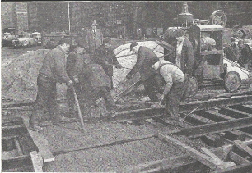
CONCRETE is being poured by a construction crew at Madison-Wacker to restore the Madison street carline tracks to their original route. Temporary run-around tracks had been installed at this location on August 20, 1951, to make way for the construction of the double-deck Wacker drive superhighway extension. John L. Ruzich , division superintendent, watches the operation from the background.
