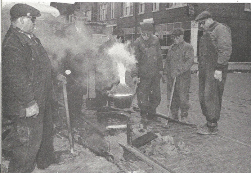
THE Thermit welding process is used by CTA for connecting rail ends to form a continuous rail and eliminate joints. These rails are preheated to a temperature of 1650 degrees Fahrenheit, determined accurately by an instrument called a Pyrometer. When the desired temperature is reached, the Thermit mixture is placed over the mold, ignited, and then poured. One of the three CTA Thermit welding crews recently completed a job at 53rd and Halsted streets. Shown here is the crew as they watch Foreman John Stiglich about to pour the mixture. At his left, holding the Pyrometer, is Joseph S. Ruzich , general foreman in charge of welding.
