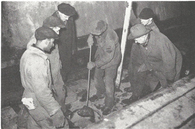
FORCES of the Rapid Transit section rodding sewers in the subway. This work is necessary in order that the sewers will function properly. Martin V. Duffy , assistant superintendent, right foreground, and Samuel Frase , track foreman, third from left, watch a workman remove a large piece of concrete which evidently had fallen into the sewer when the subway was under construction. After sewers are cleaned they are thoroughly flushed out with water under pressure.
