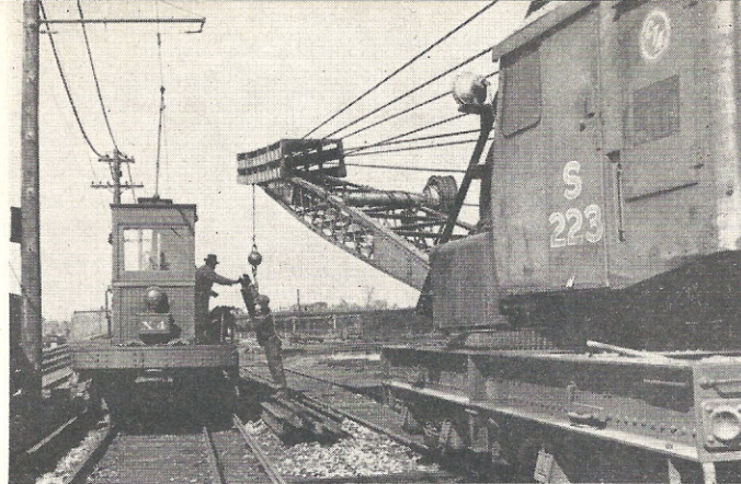
LABOR-SAVING devices save a good many back aches in the material yard at 313 East 63rd Street. A laborer in the yard, center, is guiding a rail being swung from the stockpile with a mobile crane to Peter Mirkovich , frog shop foreman, who had come into the yard with a work car to pick up needed material.
