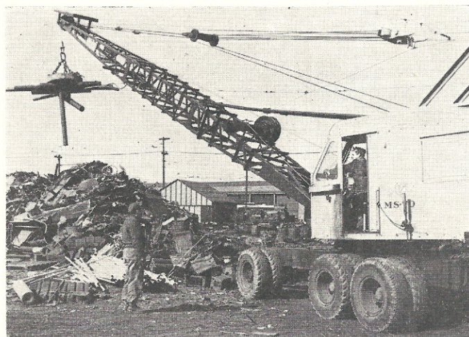
MATERIAL and Supplies workers accumulate and grade each years thousands of tons of scrap material to be sold to the highest bidder. Working on the scrap pile in the South Shops yards, with the help of a rubber-tired crane and a huge magnet, are Eddie De Stefano , crane operator, and his helper, Bill Gerber .
