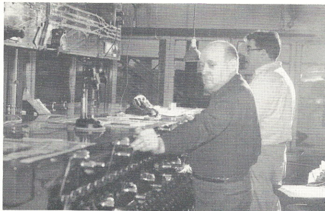
ALL Rapid Transit (elevated-subway) train movements are controlled by Transportation Department towermen located at various strategic points on the system. Louis T. Peterson , foreground, and James H. McManus are shown operating the model board controls at the Howard Street terminal where 105 train movements per hour occur during rush periods.
