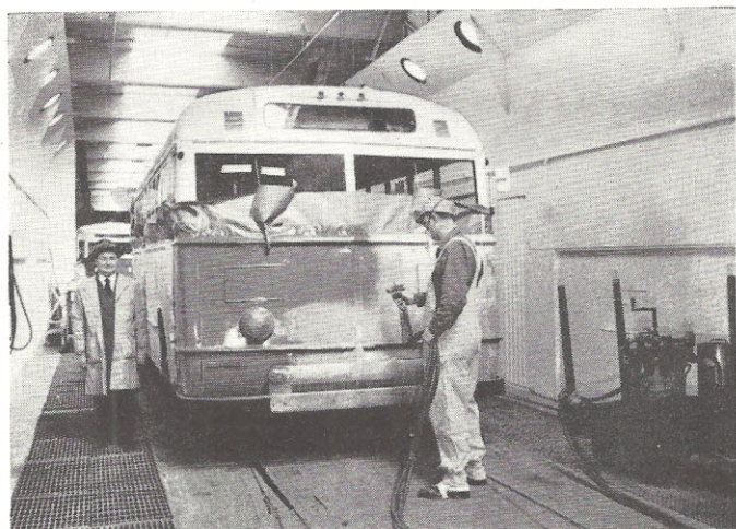
ONE OF the brightest spots in the West Shops because of the strong lighting used is the spray booth in the paint shop. John Danloe , foreman (left), stands by as Elray G. Blake , painter, applies coat of Everglade Green hot spray paint to lower body portion of Ford 25-passenger bus. Croydon Cream paint has already been sprayed on the upper half.
