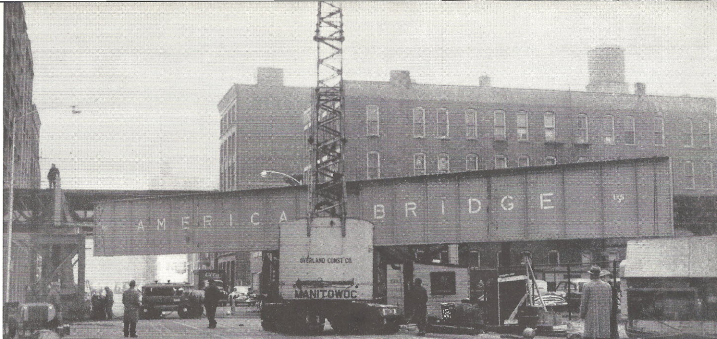
INSTALLATION of new 86-foot plate girders spanning Ontario street at Franklin street was in progress when this
