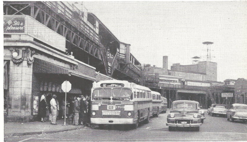
HEAVIEST transfer point on the CTA system outside of the Loop proper is the Logan Square terminal, where passengers transfer between the Milwaukee avenue “L”-subway route and buses serving wide areas on the northwest side. Direct transfer can be made to five surface routes at this station. These are Milwaukee avenue local and express buses, Kedzie-Homan buses, Kimball and Logan-Diversey buses.
