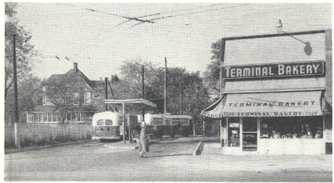
THIS OFF-STREET facility at Grand and Nordica (7000 W) serves as the western terminal of the Grand avenue route. It was established in 1951 and is one of 101 such facilities on the CTA surface system.
