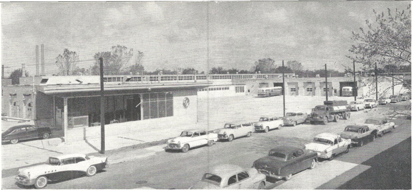
GENERAL VIEW of Forest Glen bus terminal's service building is shown in this picture which was, as were the other pictures, taken during the latter stages of construction. In left foreground is the service area equipped with four undershelter
