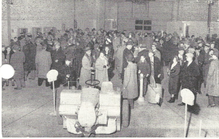
CONVERGING AT EAST END of repair area around refreshment tables is part of the estimated 3,500 visitors who attended the open house. The crowd was one of the largest ever present at an open house of a new station.
