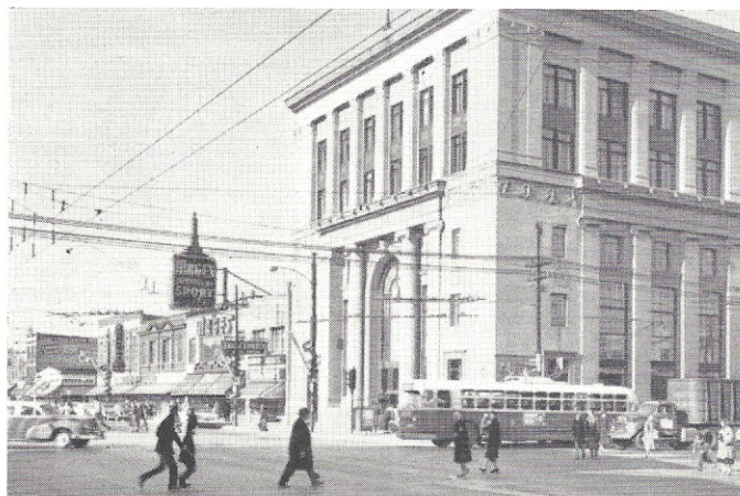
TYPICAL of the transfer points around which substantial outlying business districts have developed is the Pulaski-North avenue intersection, shown here.
