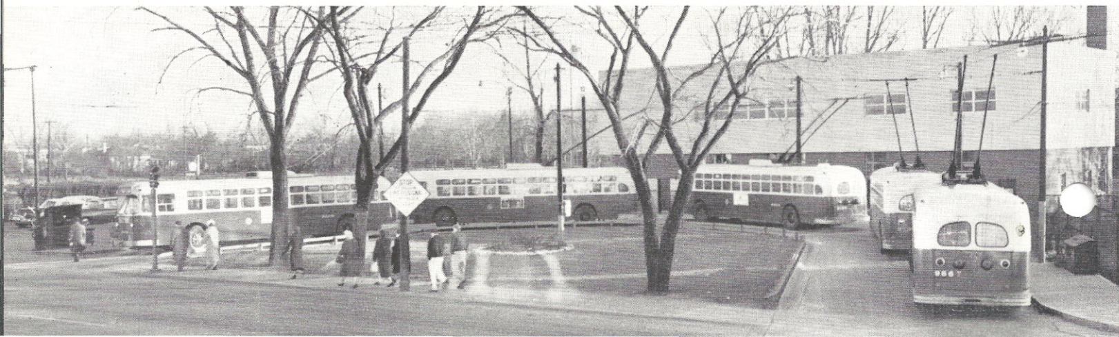
MORE THAN 100 off-street facilities such as this serve as terminal points for CTA surface system routes. Pulaski trolley buses have been using this turn-around at Peterson road since 1951.
