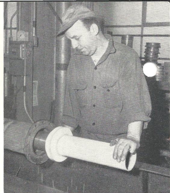
CAREFULLY POSITIONING tool, similar in appearance to a section of pipe, Machinist Charles Dreasler makes sure he aligns axle housing tube with the ring gear housing.
